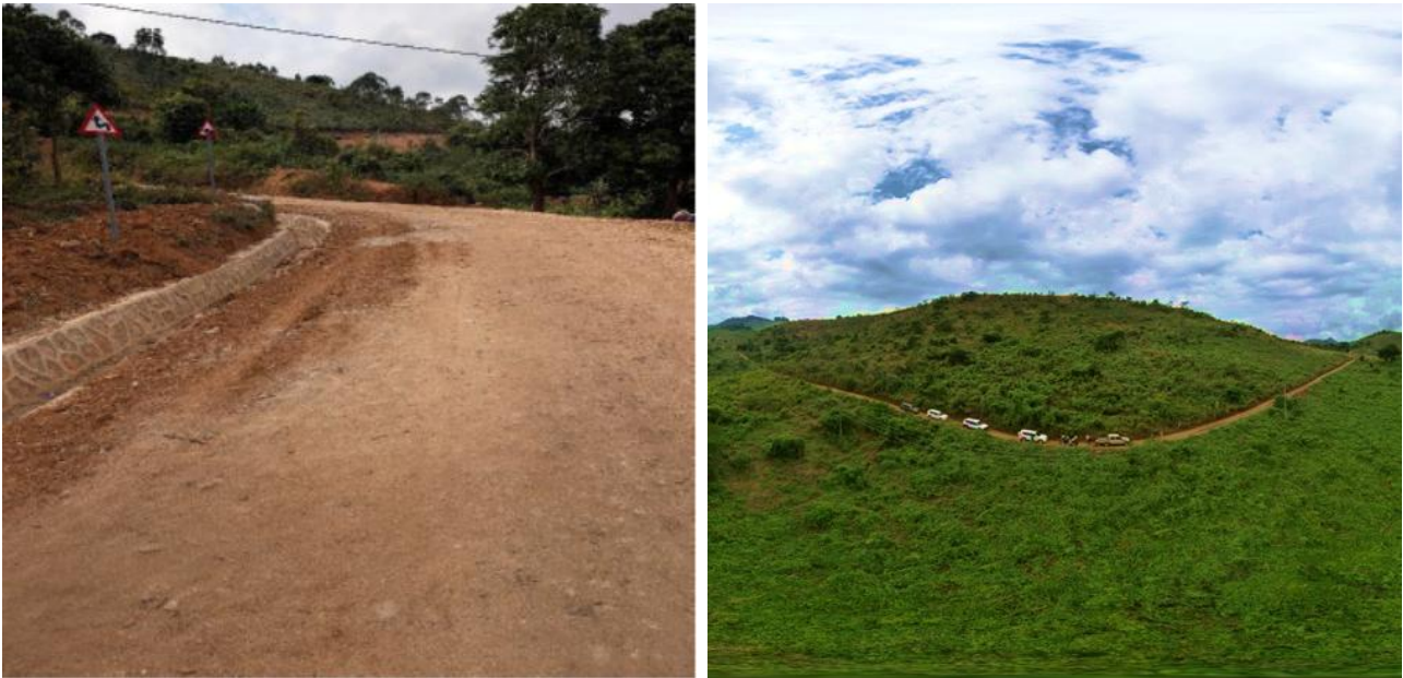
Figure 1 – Southern Access Road
